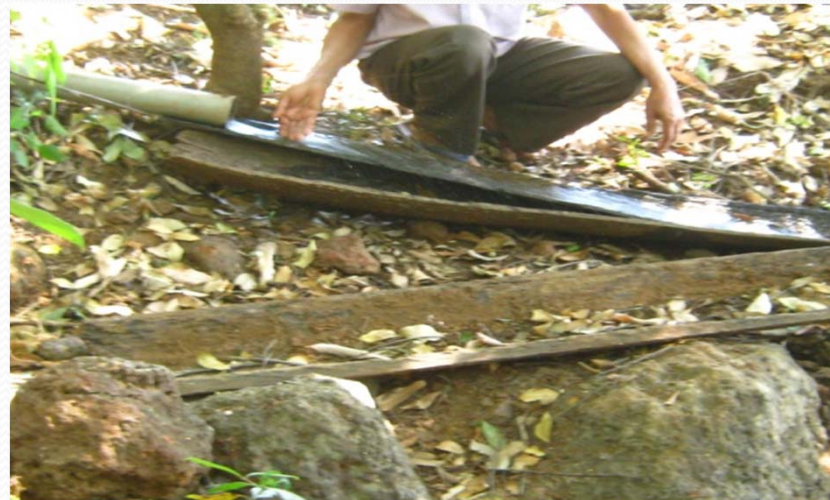
Natural Stream water collected through PVC - Pipes and Wooden Flakes
